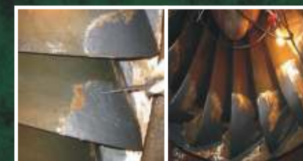
Anti-abrasion coating Rebuilding of hydroelectric plant
